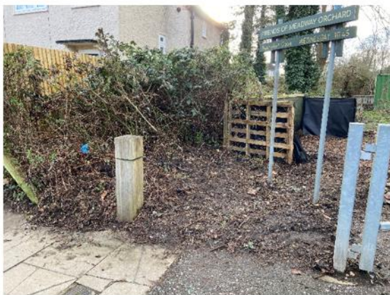
Area cleared for new sign to go in
