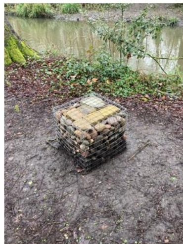
Gabion for single seat, with stones. The wooden bench still needs to be secured
