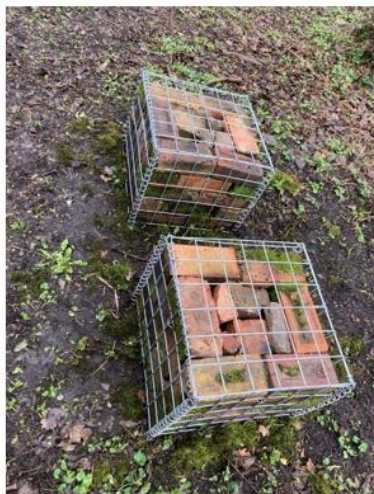
New gabions installed as seating on the island. The bricks were sourced locally and the wooden bench on top still needs to be secured.
