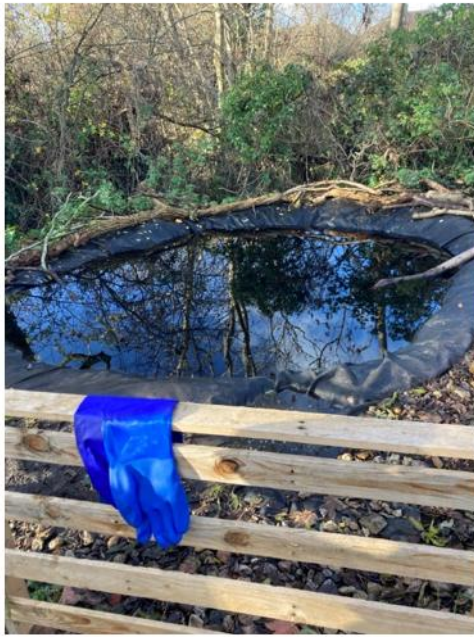
New pond in Meadway Orchard, dug by hand, with logs from surrounding areas
