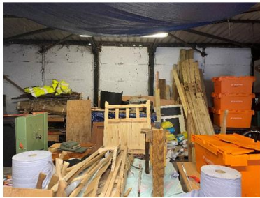
Image 1: Wall intended for the plywood backing. Holes between the roof and wall visible.
