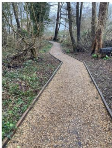
New paths in Crane Park Island, funded by the previous Crane Valley Community Fund.
