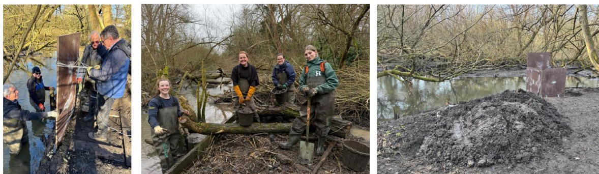
Left: Ian from FORCE and other TCV volunteers installing the front panel of the kingfisher bank
