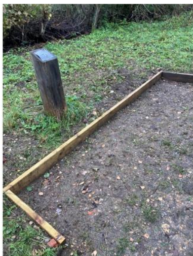
Image of new wooden sleepers installed at Crane Park Island, ready for the new shingle to be placed. One of the metal plates can also be seen in the background
