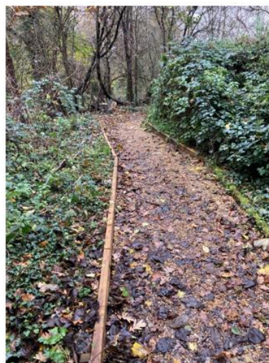
Image of new gravel paths with wooden sleepers installed at Crane Park Island
